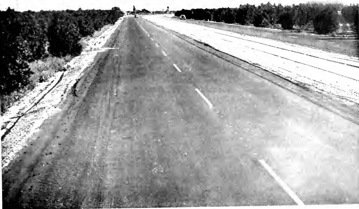
At top—View of realigned portion of State Highway Route 77, including a suggested intersection point indicated by striped triangular traffic island. At bottom—View of 4-lane section through orange orchards.
